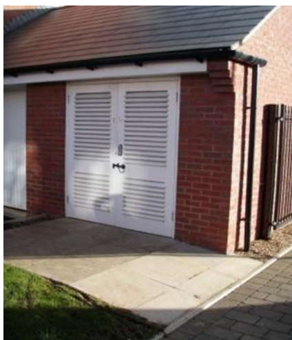
Ideal communal bin store with adequate storage, ventilation, security and access.
