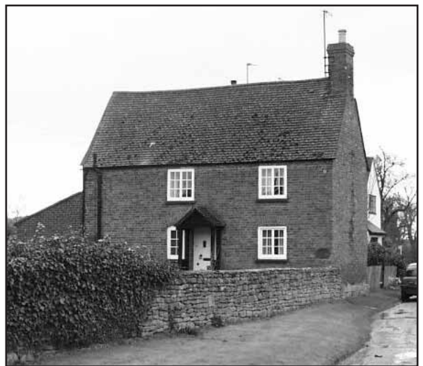
School House and its dry stone wall
