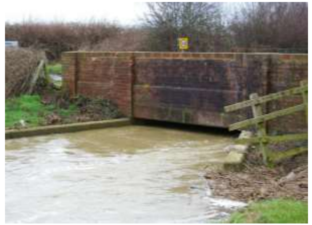
Down Hatherley Bridge, Frogfurlong Lane, January 2008
