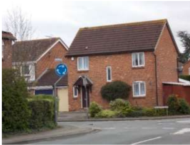
Variegated brick used in new build at Pirton Meadow
