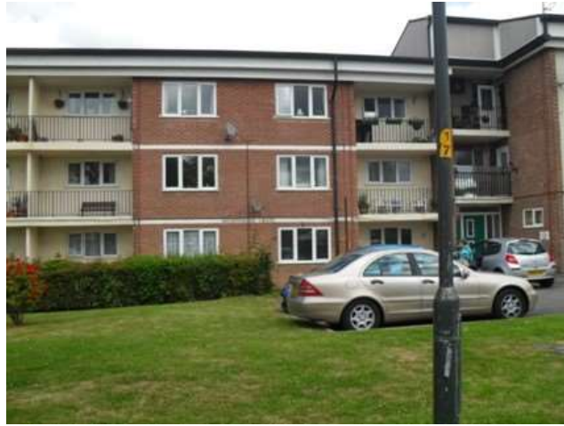
Mix of brick and render, Nightingale Croft (Severn Vale Housing Association)
