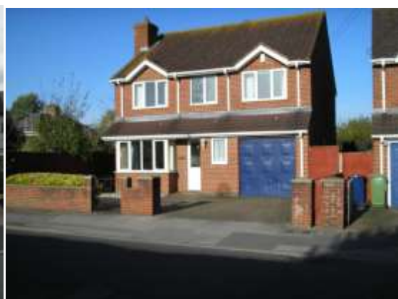
Modern House, Morley Avenue
