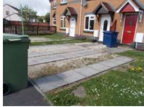
Highgrove Estate, Churchdown (good space provision for cars but inadequate hardstanding materials)
