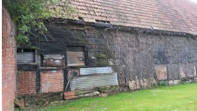
Elm boarding on farm building at Pirton Court, Pirton Lane (credit: R Warne)
